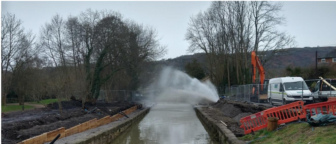
Figure 2: The second water main bursting and spraying water.
